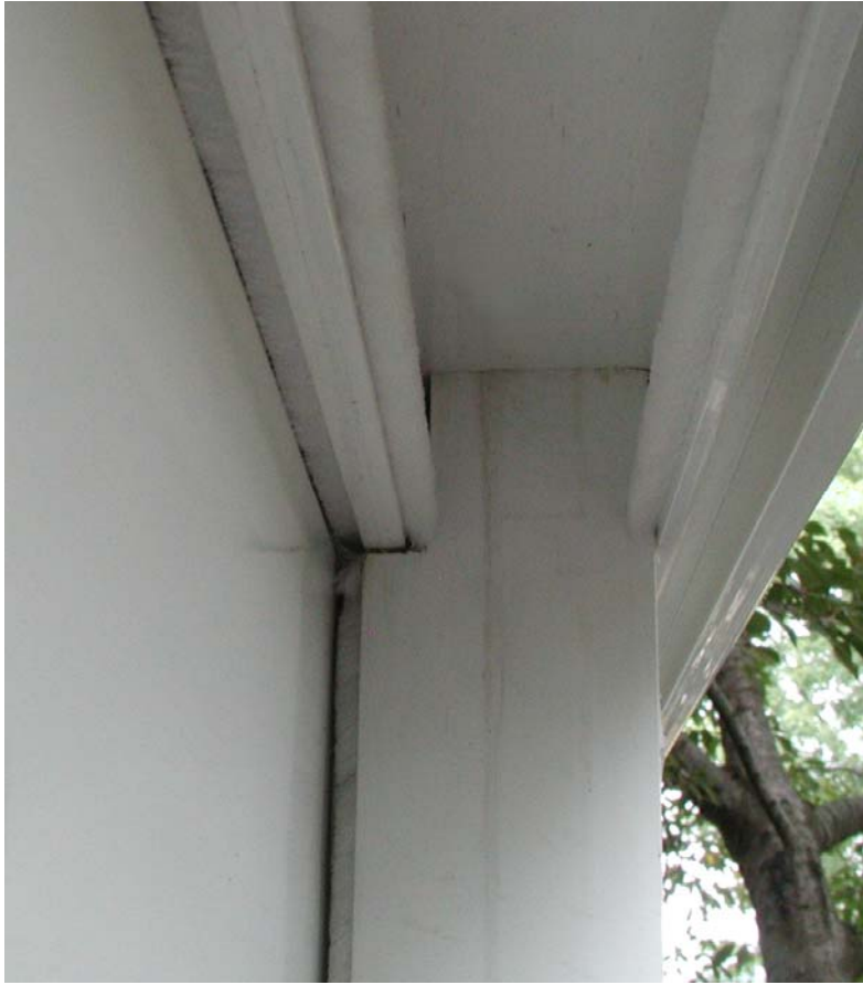
Head end of interlock panel.
