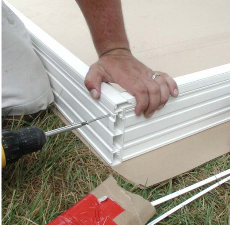
Attach head to right and left jambs.
