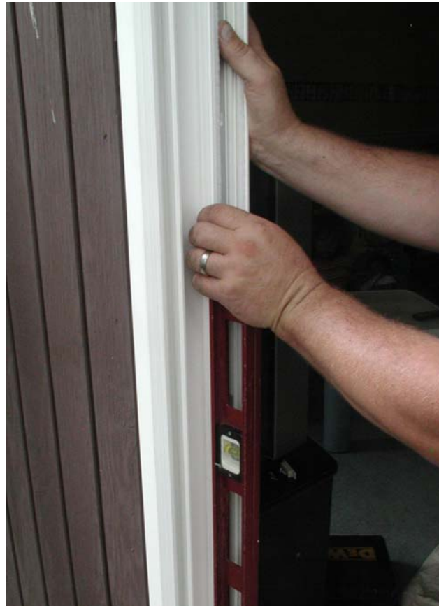
Check jamb for level.
