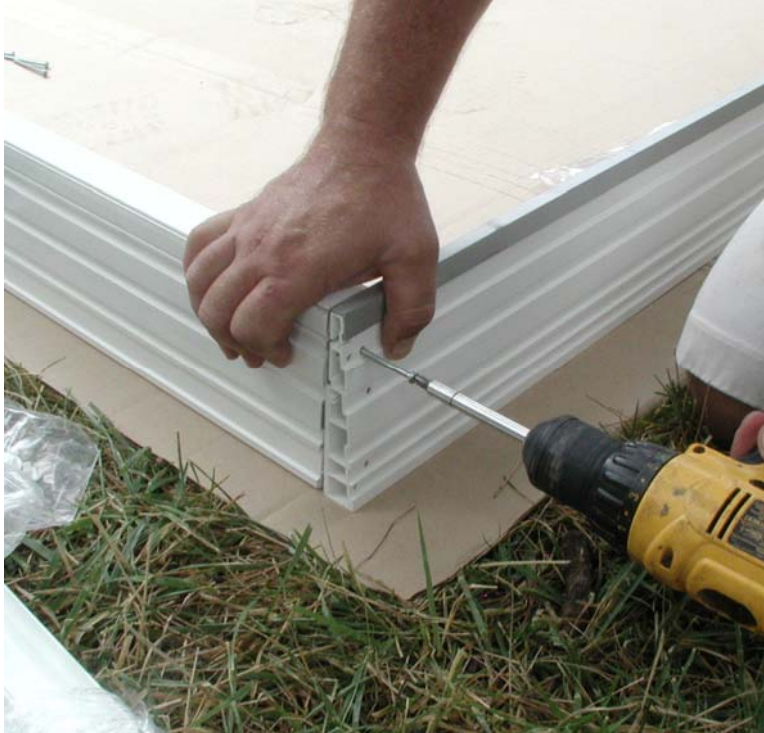
Attach sill to right jamb.
