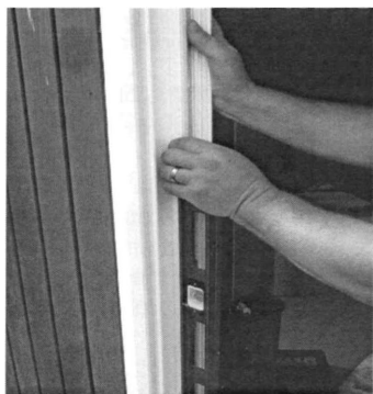
Check jamb for level.
