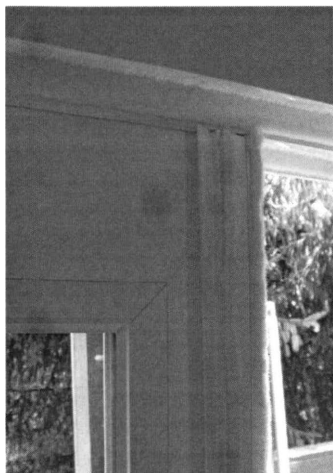
Check for gap at top of Interlock
