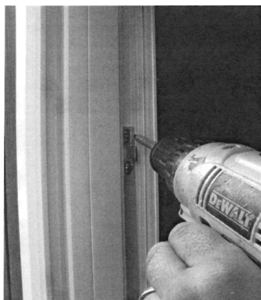
Keeper adjustment
